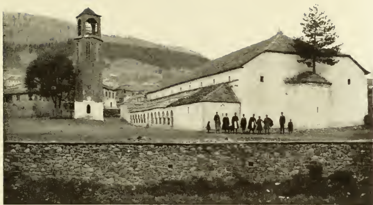
1. EXTERIOR FROM THE EAST
